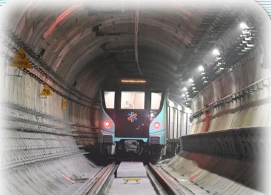
Colaba-Bandra-SEEPZ (Mumbai Metro Line-3)
