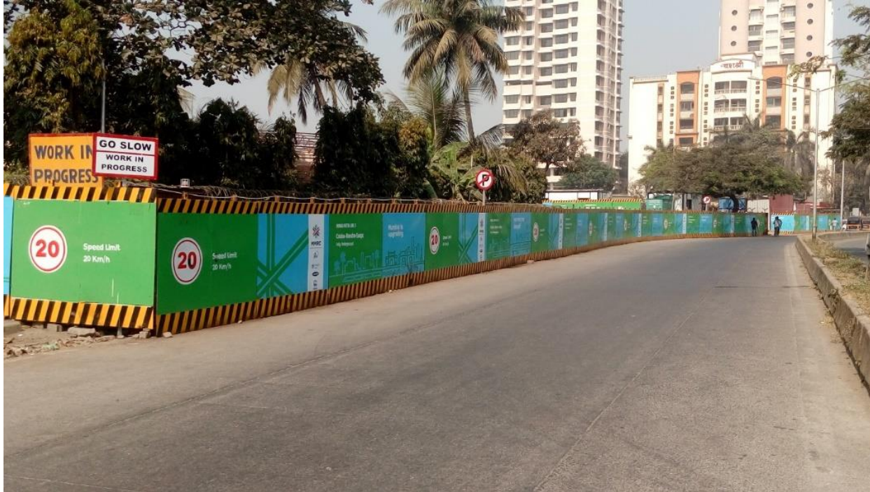
Enclosed work areas
