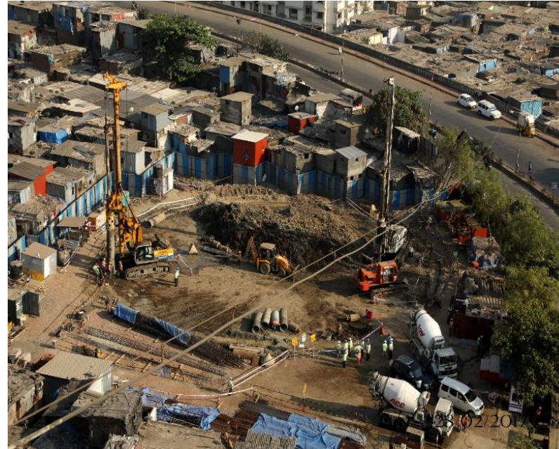
Site After Demolition
