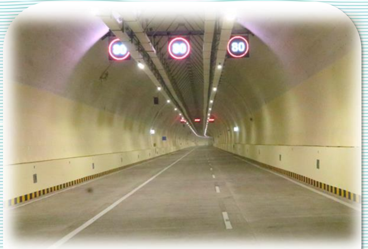
Mumbai Coastal Road Project (South)
