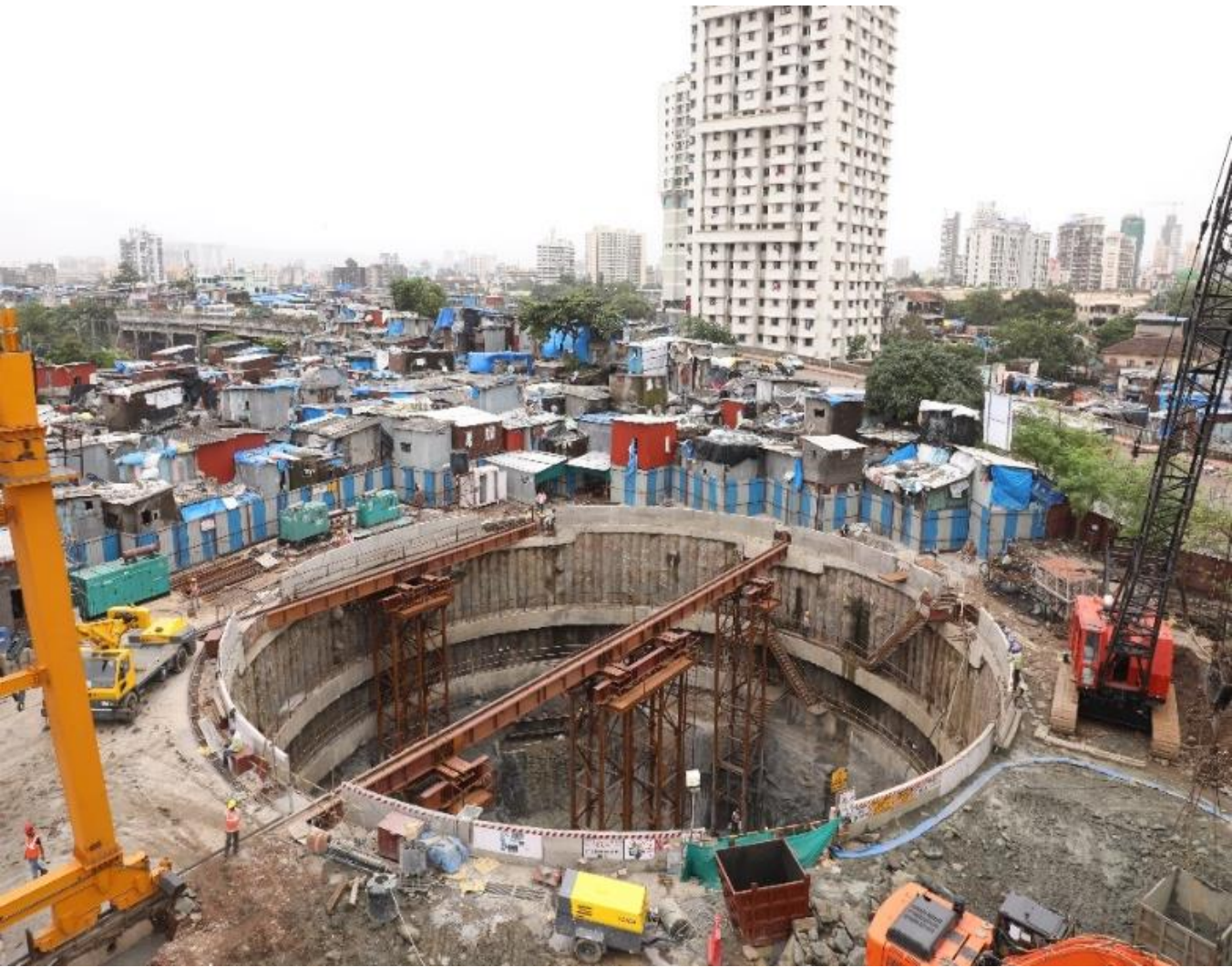
TBM Launching Shaft & Lowering of TBM
